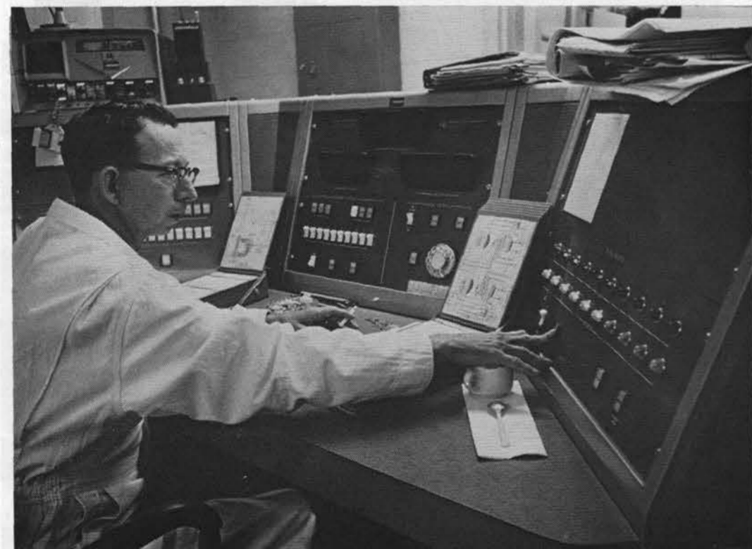
WITH THE TOUCH OF A FINGERTIP, James C. Vincent (4511) can check the operation of heating and air conditioning equipment in any major building at Sandia Laboratory. The monitor and control console is manned around the clock. Operator can contact maintenance man in the area by radio to take care of any malfunction in buildings.
